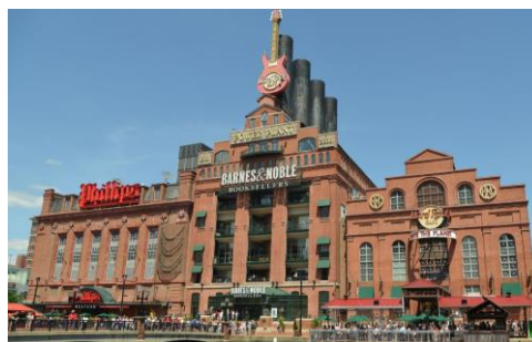
Pratt Street Power Plant
